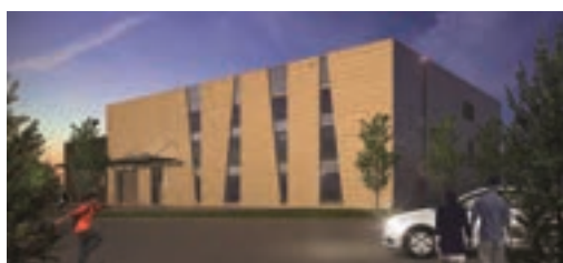
The new Shaganappi Pump Station which was completed in January 2022, has a design capacity of 220ML/d (Image courtesy of The City of Calgary)
