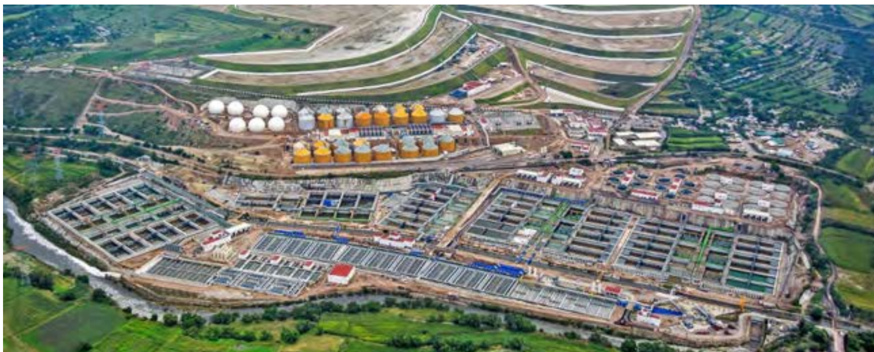
Clarification Plant, Atotonilco, Mexico
