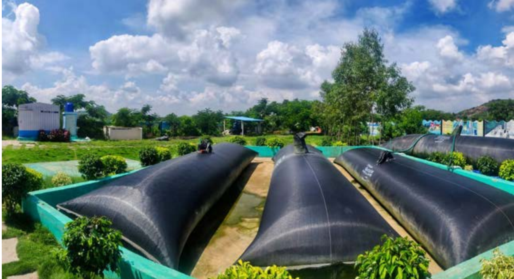
Figure 1: Panoramic/ Wide Angle Views of the FSTP
