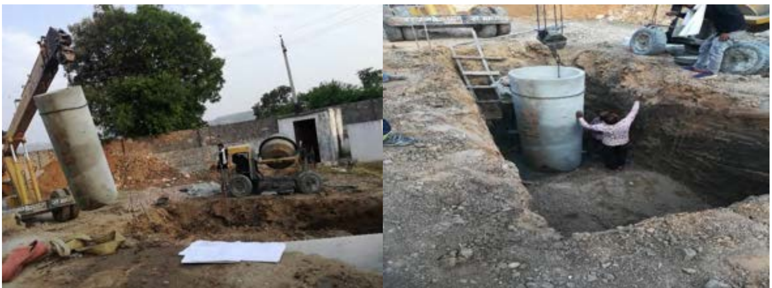
Various Stages of Construction - Part I
