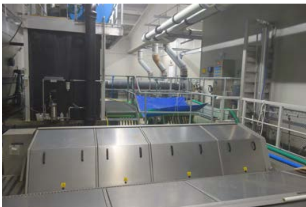
The drum filters at Swiss Alpine Fish are 3,600 millimeters long and have a diameter of 2,000 millimeters.
