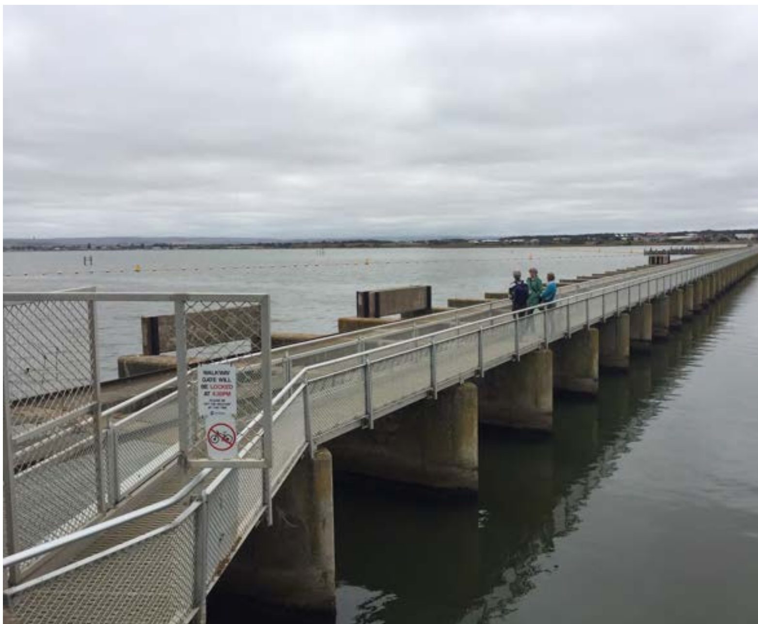
Barrages on the Murray River play a vital role in fresh water irrigation
