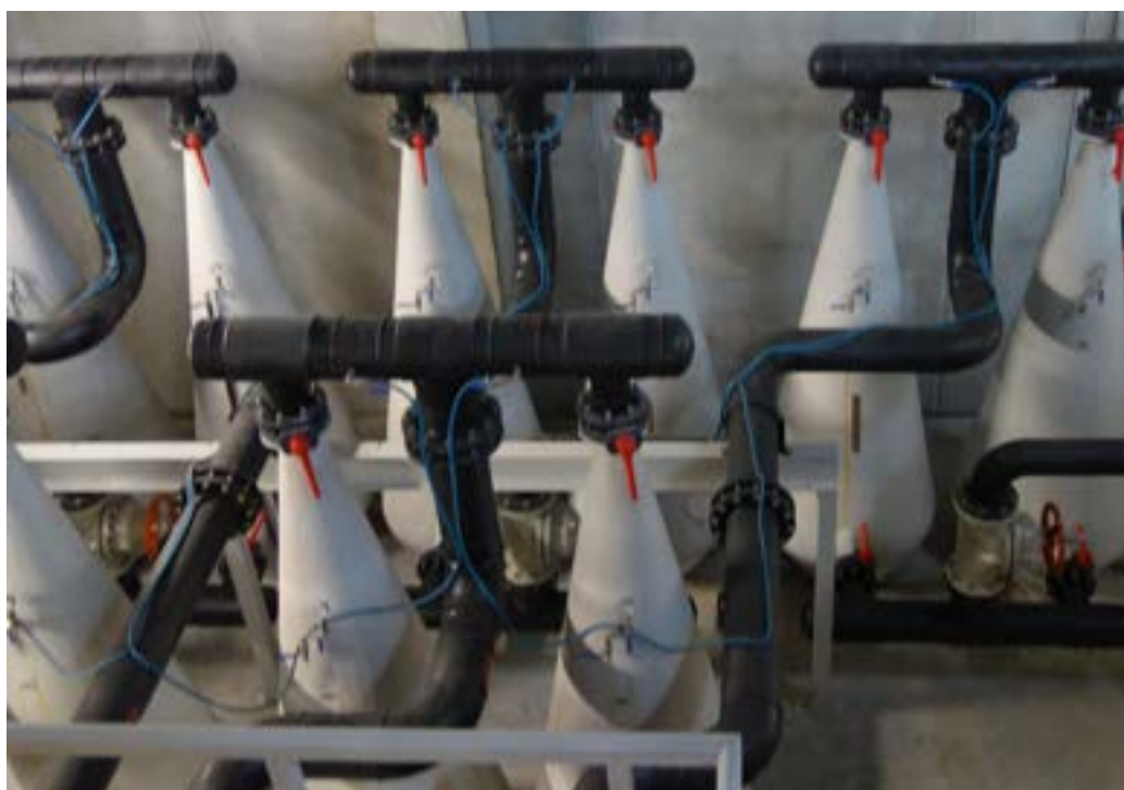
Some of the cleaned water is fed into oxygen cylinders and enriched with oxygen at a pressure of three bar.
