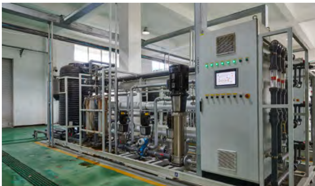
Just a few of many Grundfos pumps (these are CRN and CMs) in the WELLE membrane treatment facility.
