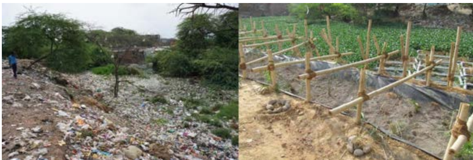
Before and After Pictures Showing Work at a Slum in Delhi (2014)
