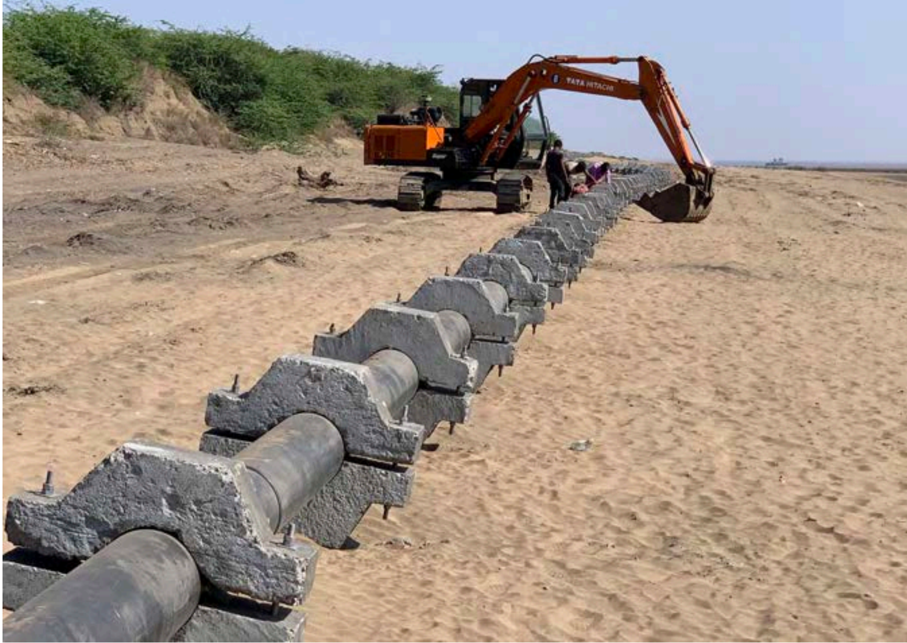
Installation of HDPE Pipeline with Concrete Sinker-Blocks to Sink and Secure the Pipeline in the Sea
