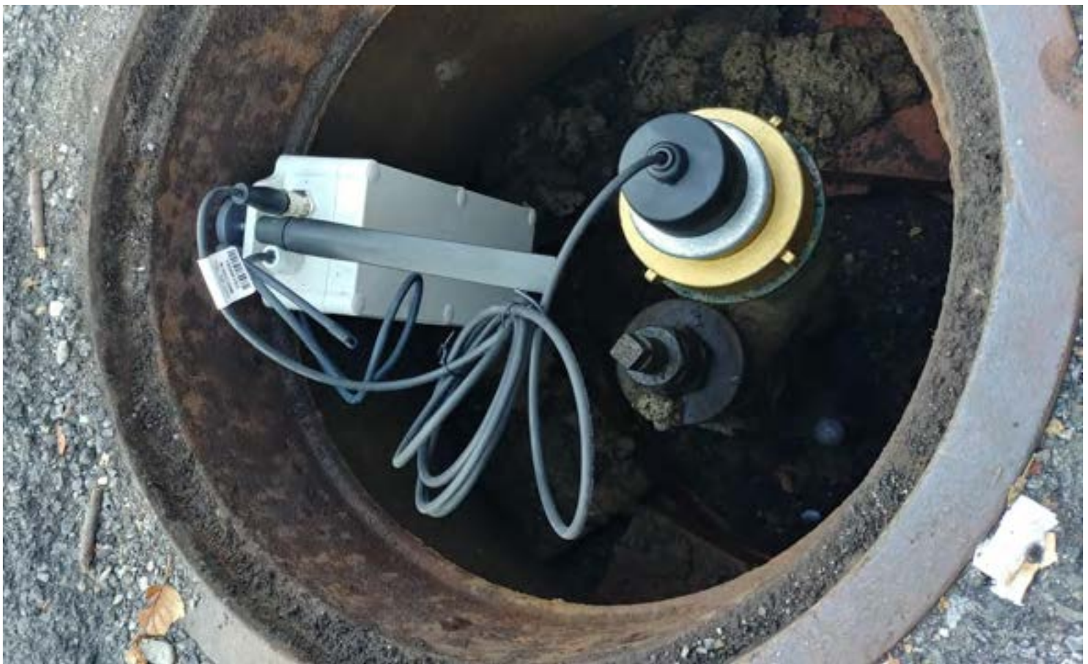
Figure 2 B: AQS Underground Acoustic Sensor Installation
