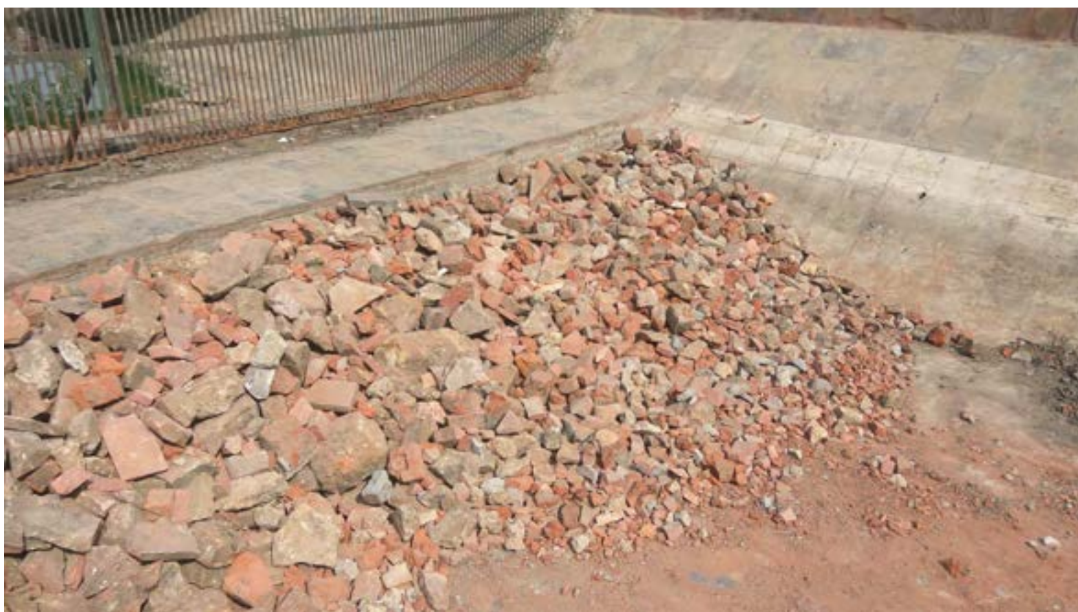
The Start of the Wetland in the Inlet Channel
