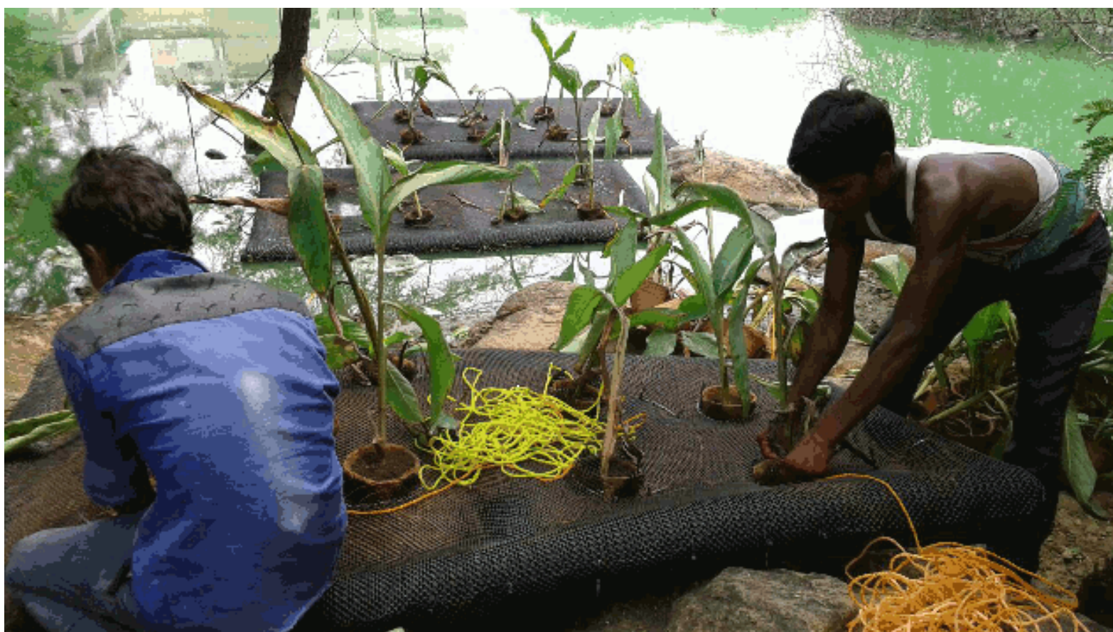
Making and Launching Floating Wetlands
