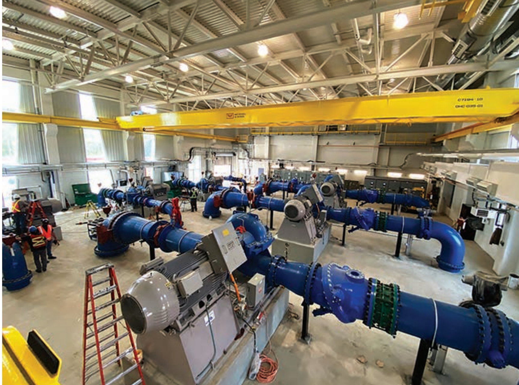
The requirements for Shaganappi involved the supply of three large RDLO 600-600 pumps rated at 80ML/d and three smaller Omega 300-560 pumps rated at 30ML/d.
