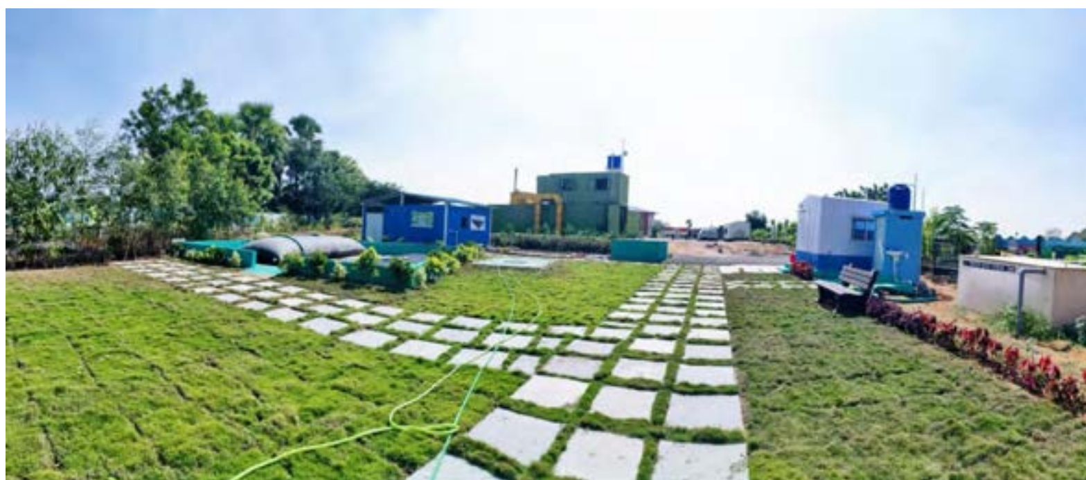
Figure 3: Panoramic/ Wide Angle Views of the FSTP
