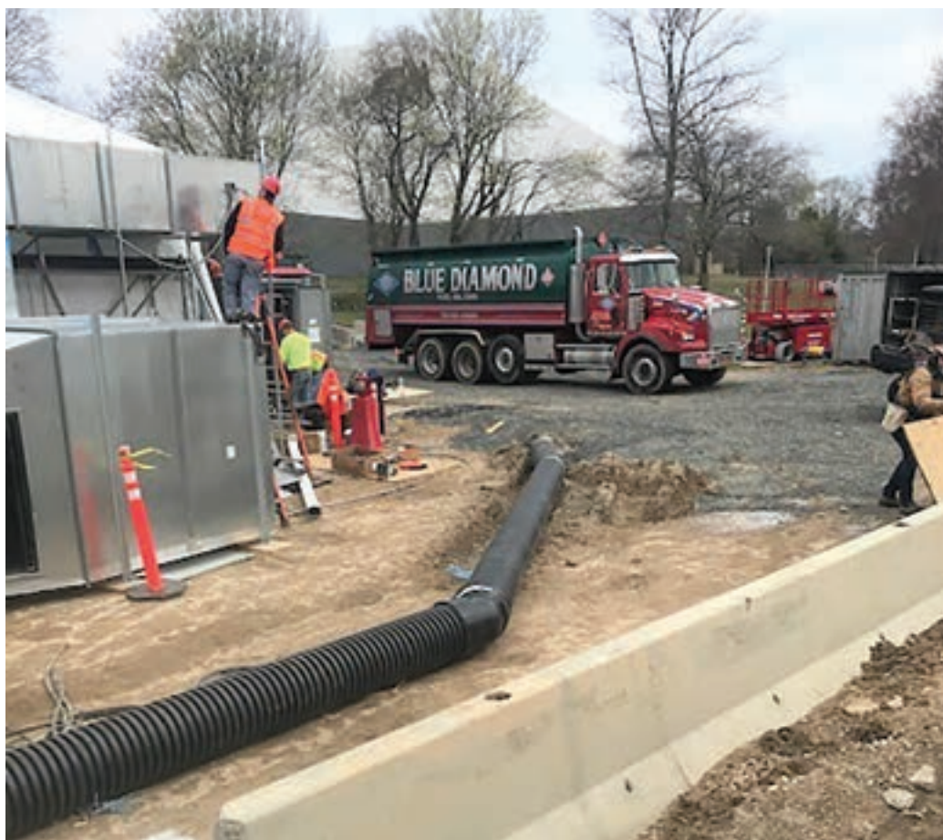
The ADS N-12 stormwater drainage pipe was run under roads and parking areas at the U.S. Army Corps of Engineers' Long Island, New York field hospitals.
