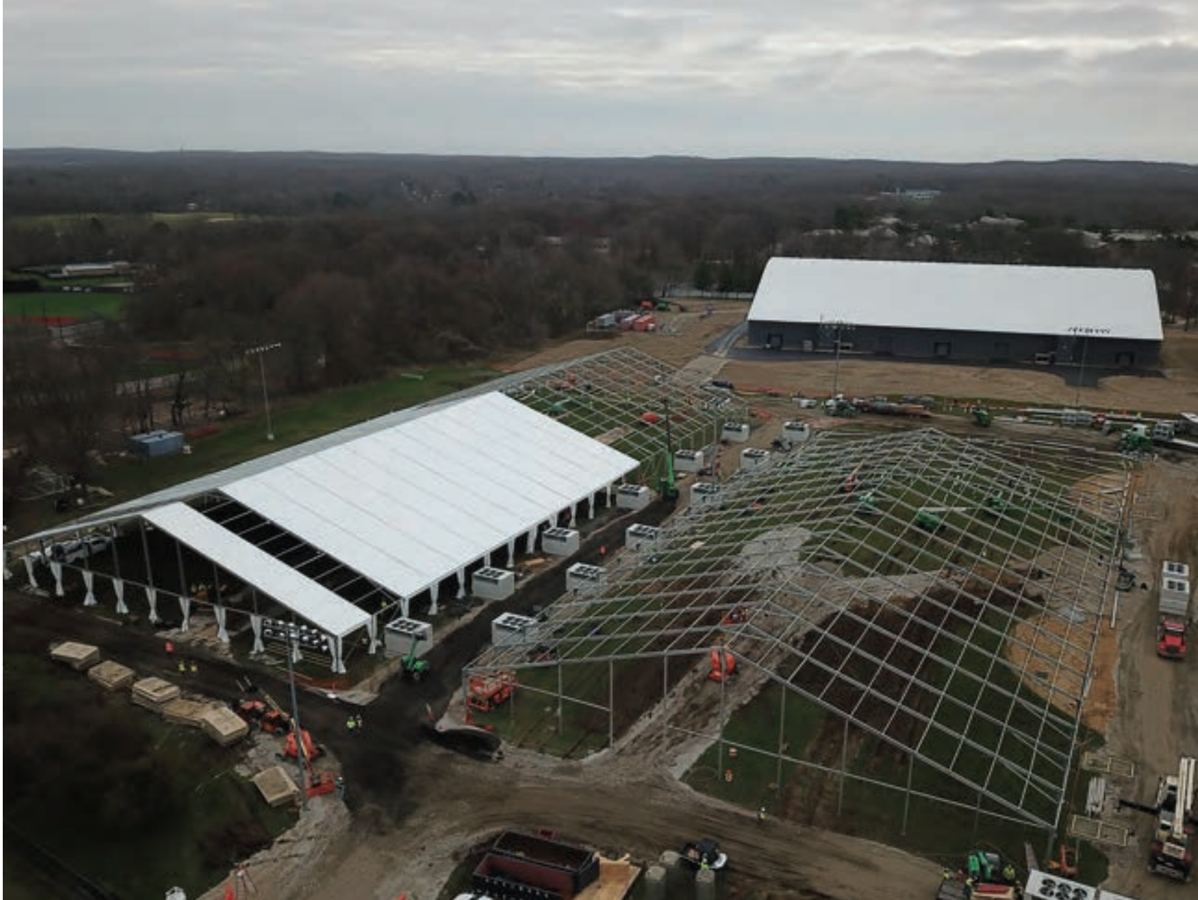
The field hospital at Stony Brook University was completed in record time. Photo by U.S. Army Corps of Engineers.
