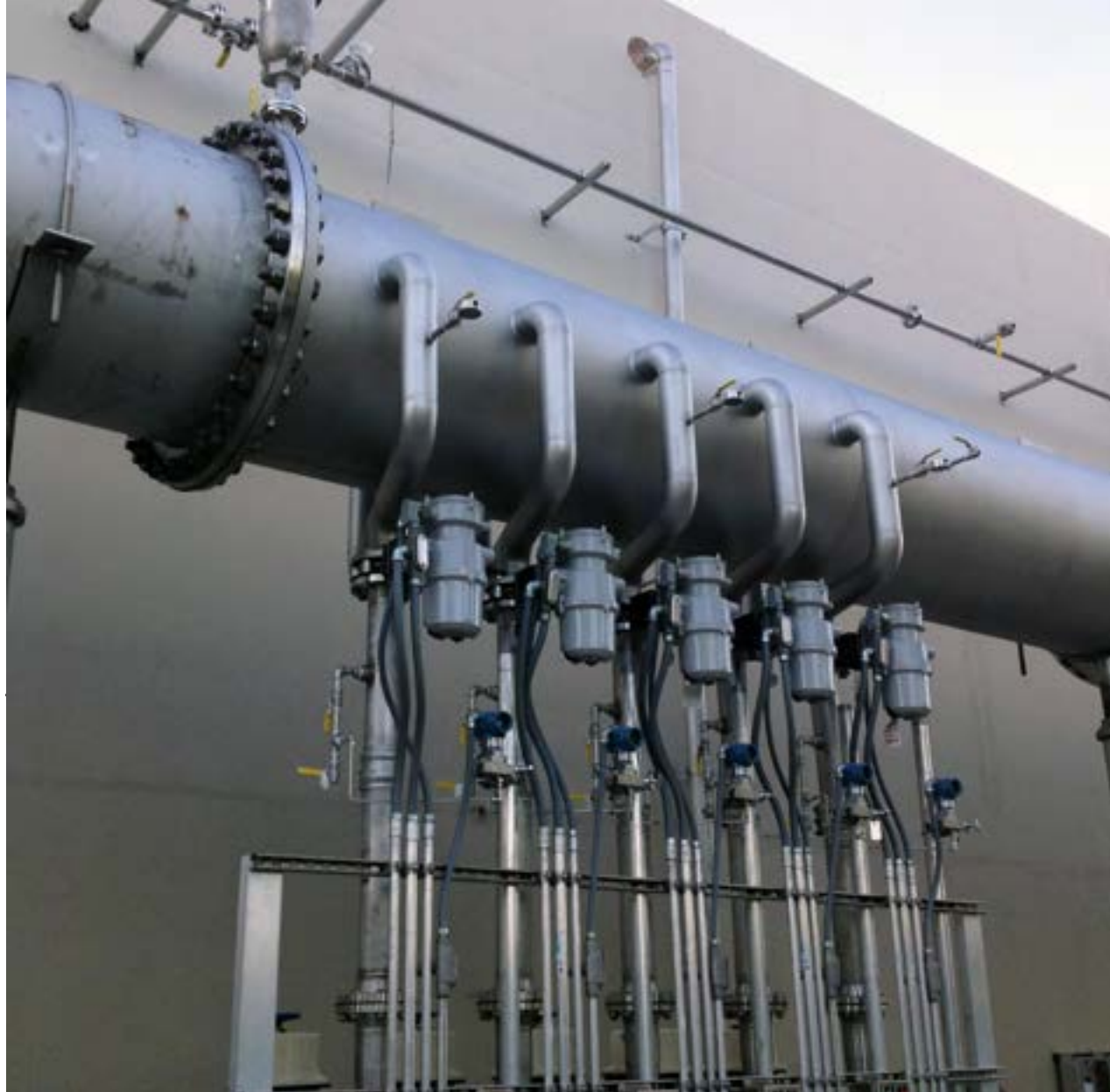
Five venturi injectors ozonate a sidestream flow and mix the treated water into the main flow in a Pipeline Flash Reactor (PFR) at OUC Southwest WTP.
