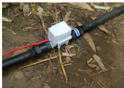
Solenoid valve installed at ground level
