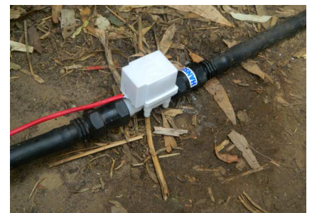
Solenoid valve installed at ground level
