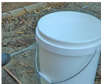
Drill a hole in the side of the evaporator
