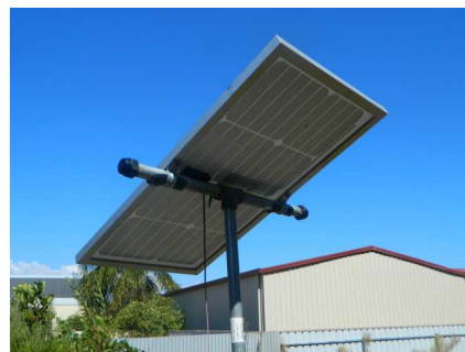
Solar panel mounted on a pole
