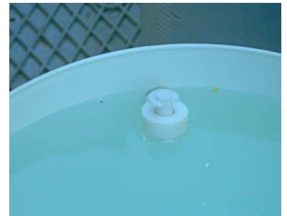
Water level just below the float switch
