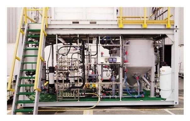
To reach the highest concentration levels with your RO brine, trust intelligent chemical softening systems like Saltworks' <u>BrineRefine</u>. Most RO systems will hit their treatment limits near 50,000 mg/L total dissolved solids (TDS). Brine Refine removes scaling ions from the water, and enables the use of <u>ultra-high pressure RO systems</u>, which can reach up to 130,000 mg/L TDS brine concentrations. Another option to maximize brine
