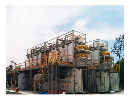
Concentrating RO brine even further requires thermal systems, such as evaporators or crystallizers. Although they cost more than RO systems, thermal systems can reduce RO brine to zero liquid discharge solids. Maximizing upstream RO recovery will minimize the size and operating cost of your thermal treatment steps.
