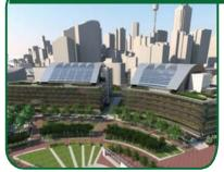
> Design, Build & Support for a Recycled Water Plant, to treat 400 kL/day of sewage (sewer mining project) for a low rise sustainable development in Zubair > Process: ECOMBBR™,
