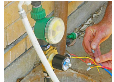
Connect the blue and green wires to the solenoid valve
