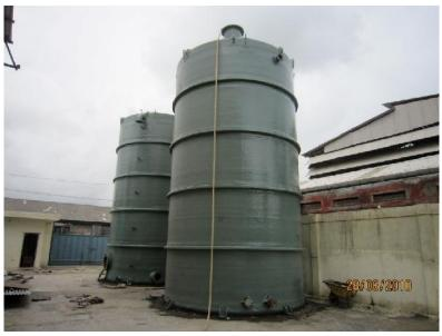
**Client :** Siemens Limited | **Equipment :** 125 m3 Sodium Hypochlorite Storage Tanks
