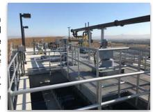
water, onsite testing evaluated both surface water reservoirs to ensure the treatment technologies chosen can meet all project goals. Kruger was selected to supply the ACTIFLO® CARB ballasted clarification system as part of the 4.5 MGD initial capacity of the WHWTP. The WHWTP is designed for future expansion to 9.0 MGD.
