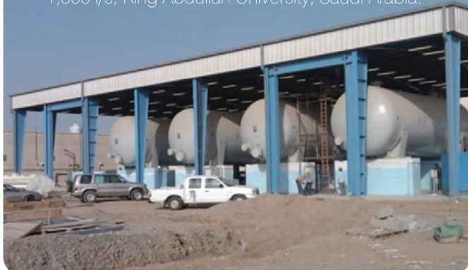
FilterClear Pre-filtration for Reverse Osmosis Desalination 1,300 l/s, King Abdullah University, Saudi Arabia.
