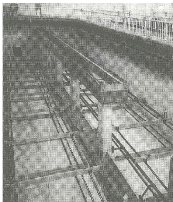
**Figure 4.9.2 Flight and Chain Sludge Collection, Figure**
