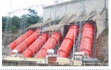
In 2012-2013, the 6 penstocks and hoist crane of the Akasombo Dam have been treated with the Zingaceram system. This system has a life expectancy of >15 years in an industrial zone with high humidity and aggressive environment.
