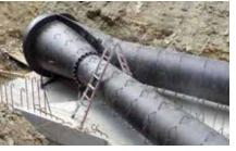
Since 2012, GUGLER Water Turbines GmbH (Austria) uses the system with Zingatarfree as a basis to protect the underground parts of water tubes. This system will provide a life expectancy of >15 years on structures immersed in soil.
