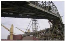
The phosphate Mine in Togo (Office Togolais des Phosphates) was treated in 1994 with 2 layers of ZINGA. In 2006 (12 years after application), no trace of rust was found. In 2014, 20 years after application, the structures were still in good condition.
