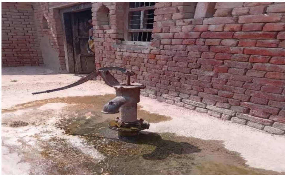
Fig. 2 | Handpump installed in houses, Nagla Chandi.
