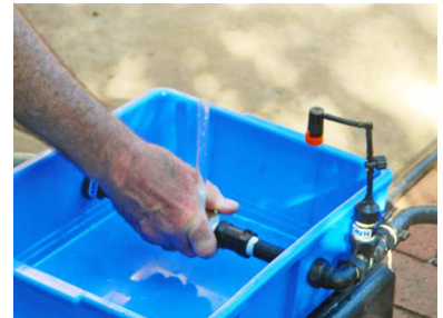
Float shaft must be vertical
