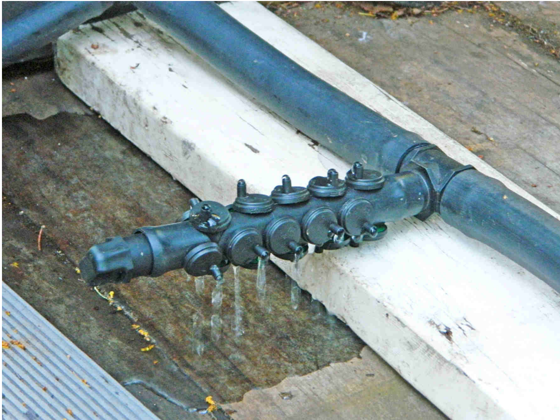
Dripper assembly with 20 drippers
