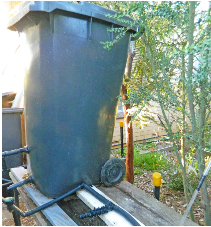
1. The header tank is an elevated wheelie bin with the top of the wheelie bin 1.3 metres above the irrigation drippers.
