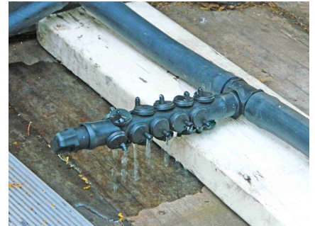
3. The dripper assembly has 20 Netafim NPC 8 lph button drippers inserted in to a short length of 19mm polypipe. The dripper assembly is connected to the 25mm polypipe.
