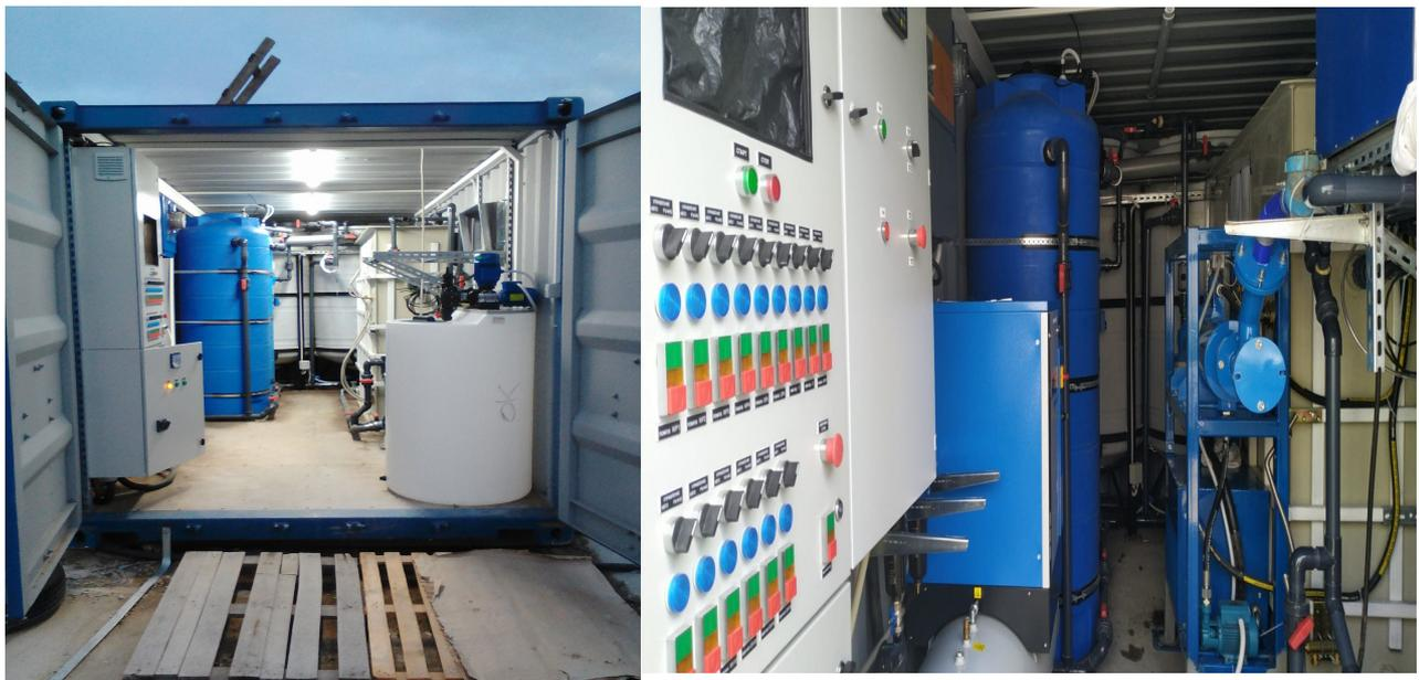
Mobile installation and equipment for wastewater treatment and sludge processing - 10m<sup>3</sup> / hour
