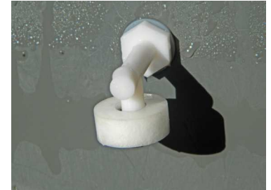
Float switch on the inside of the header tank with the float shaft pointing down
