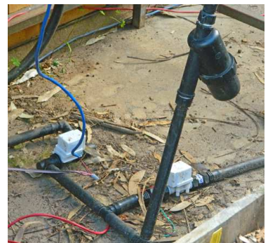
Two solenoids valves, one for each zone
