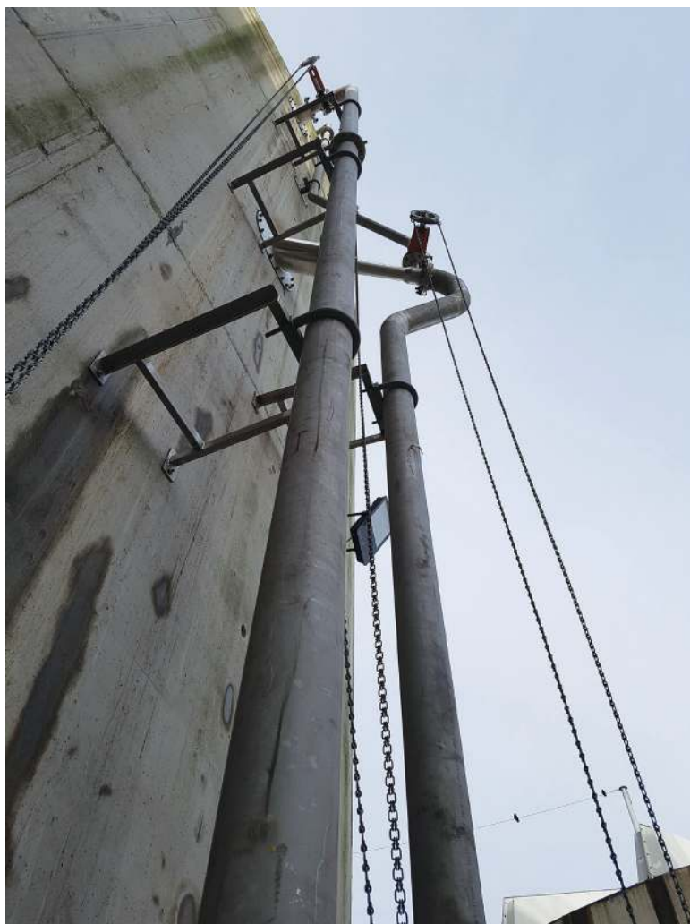
For Scottish Water, Landia's GasMix Digester Mixing System Has Helped Bring About A 25% To 30% Increase In Gas Production
