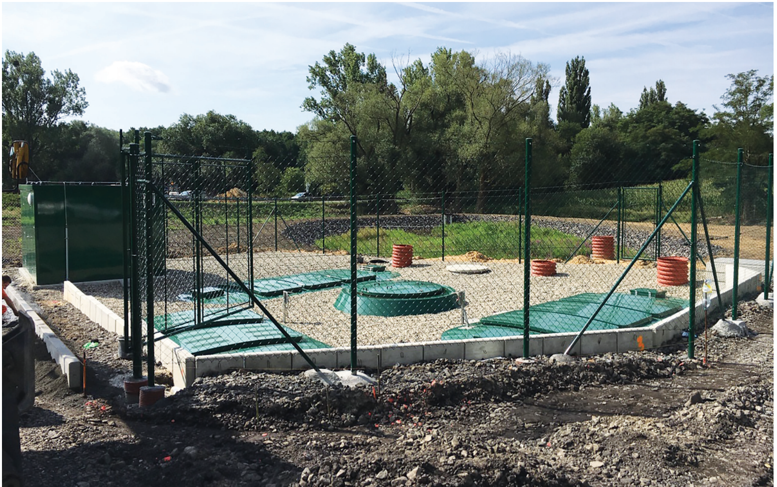
WPL's Hybrid-SAF Biological System Comprises Modular Units Controlling Chemical Oxygen Demand (COD), Biochemical Oxygen Demand (BOD) Suspended Solids, And Ammonia.
