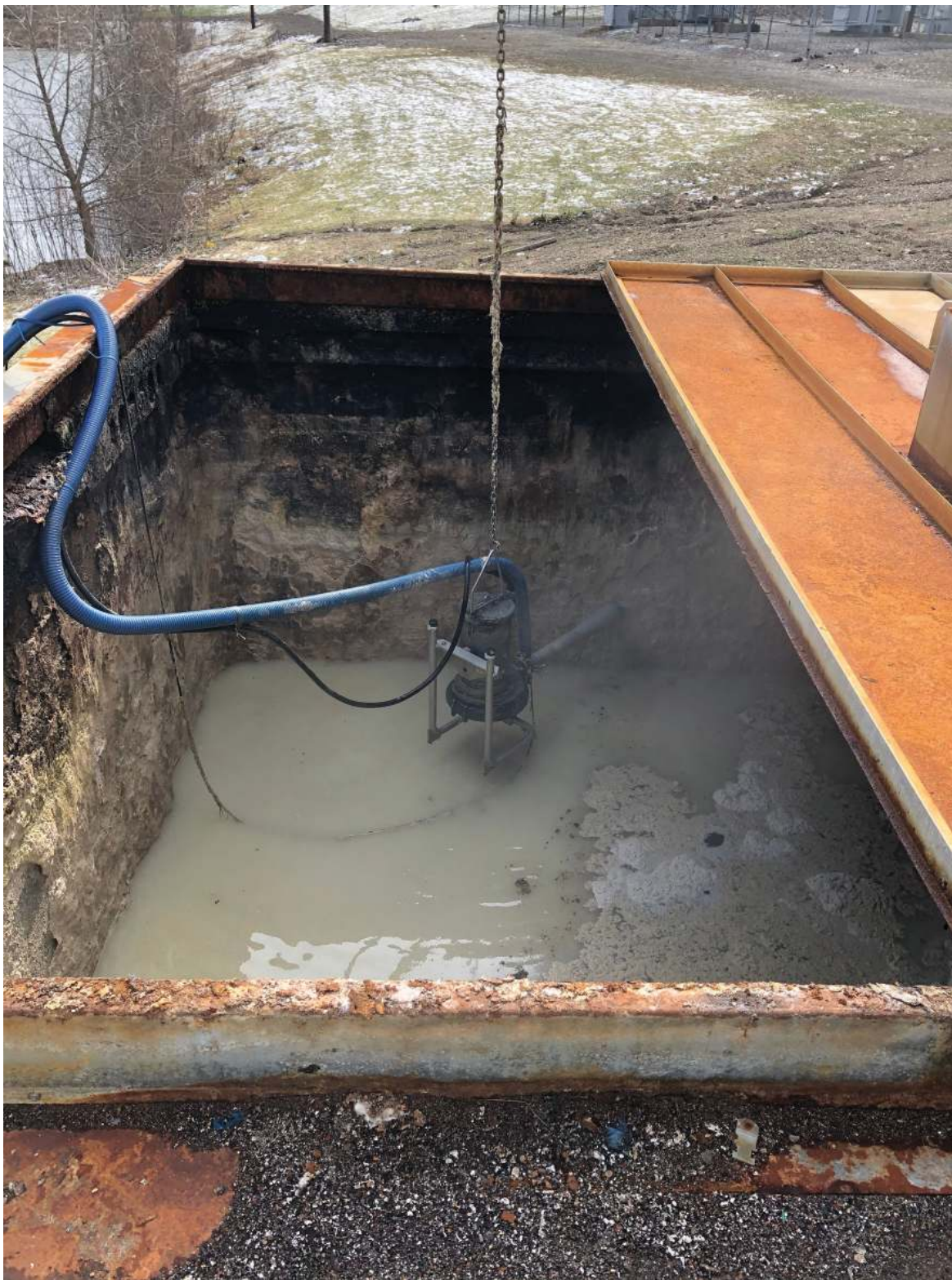
The Landia AeriGator Comprises A Venturi Nozzle And The Acclaimed Chopper Pump, Invented By Landia In 1950.
