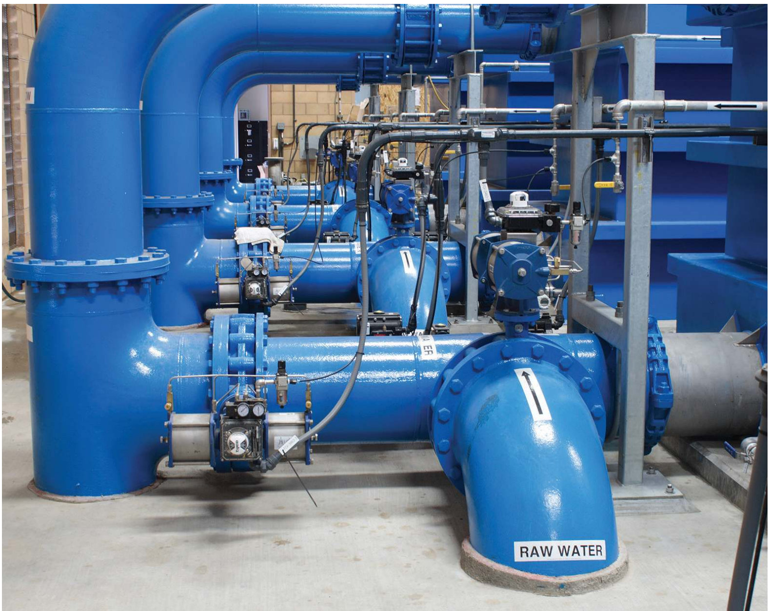
John W. North Water Treatment Plant - Membrane Filtration That Can Treat Upto 10 MGD (Million Gallons Per Day)
