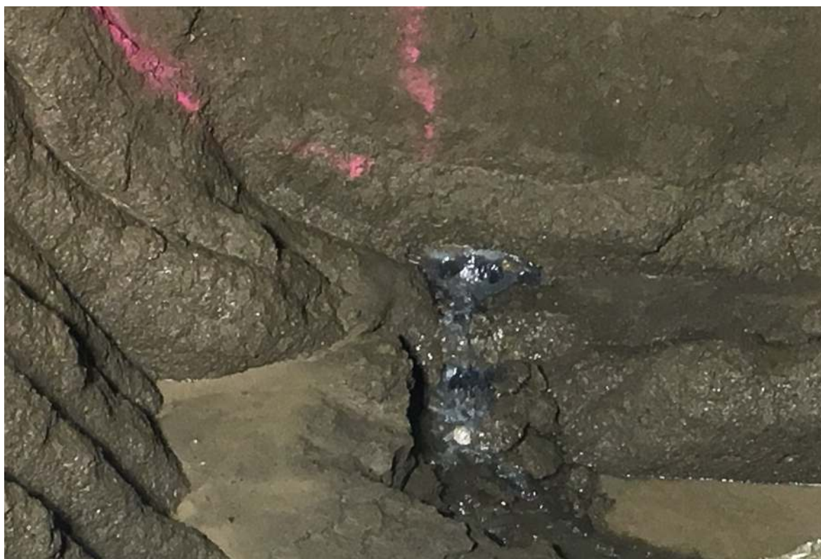
Excavation Activity Confirmed The Location Of The Leak After It Was Identified And Correlated Using LeakFinderST
