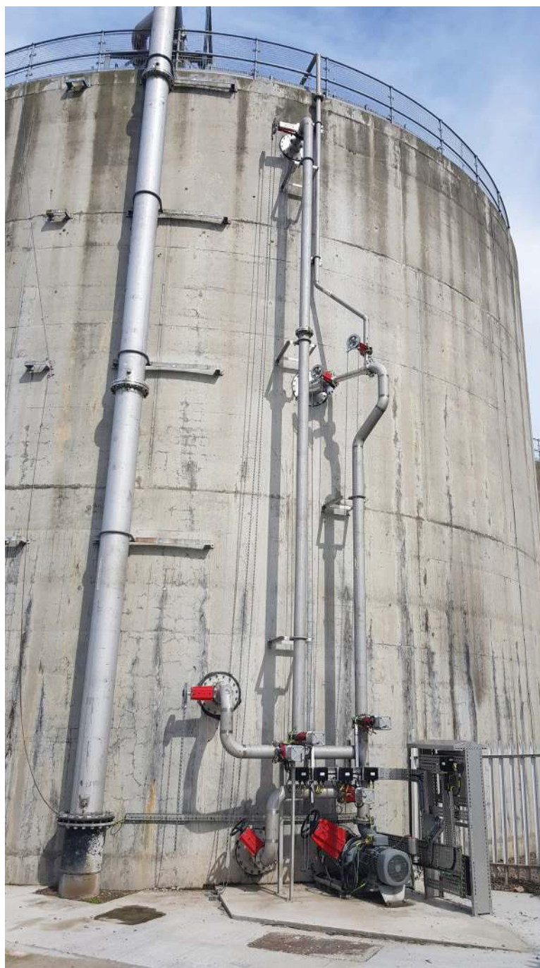
The Externally Mounted Landia GasMix At Sludge Treatment Centre (STC) In Nigg
