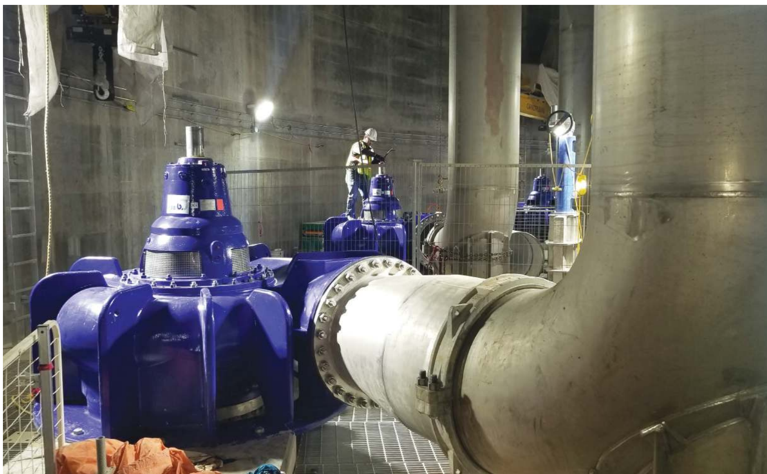
Figure 3: The First of the Pumps Being Installed and Anchored to Their Mountings (Image Courtesy of KSB Canada)
