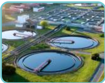
Primary and Secondary Settling
