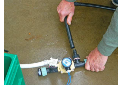
Connect the outlet from the solenoid valve to the irrigation system
