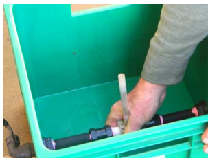
Adjust the float shaft so that it is vertical
