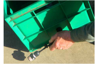
Attach the inlet assembly to the inlet pipe
