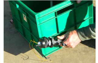
Attach the float switch assembly to the outlet pipe
