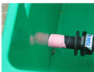
Wrap teflon tape around the inlet and outlet pipe
