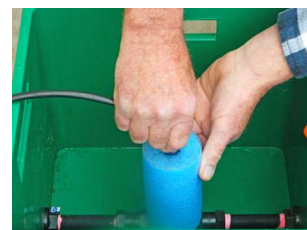
Connect the overflow tube to the top of the float shaft
