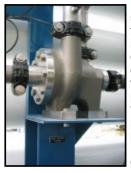
Energy Recovery — This feature saves power by recovering energy from the high pressure brine exiting the system. The energy recovery option consists of a HPB energy recovery device (ERD) from FEDCO. Energy from brine pressure turns a turbine to boost the pressure of the feed water as it exits the discharge of the high pressure pump. The FEDCO HBP is capable of achieving 80% energy transfer efficiency.
