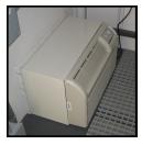
Variable Frequency Drive (VFD) — The high pressure pump is equipped with a variable speed drive (VFD) allowing the pump to operate at a proper speed. This prolongs the life of the pump and allows for soft starts and stops.
