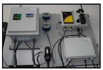
of optional analyzers can be provided to assist the client in monitoring the quality of both inlet and outlet of the system. Optional instruments include pH, ORP, chlorine, turbidity, and silt density index.
