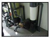
Raised Floor — The system is equipped with a raised floor consisting of fiberglass grating supported six inches above the container floor. This protects the floor of the container and provides a neat and safe environment inside the container since
