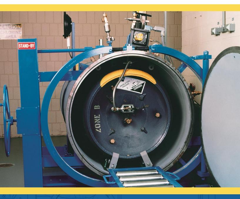
ChlorTainer is a high-pressure containment vessel into which a ton chlorine gas cylinder is processed. If the cylinder should leak, all chlorine gas is contained within the vessel and processed at a normal rate, so no hazardous waste is generated. Scrubber systems, fans, pumps, tanks, and mechanical systems are not required. ChlorTainer addresses RMP considerations, enhances site security, and provides fail-safe protection for plant operators.
