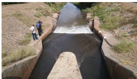
Figure 7 — Geo-localized benchmarks (in white on the left and on the right) used to measure water level, surface velocity and discharge in the Themu River Basin, United Republic of Tanzania
