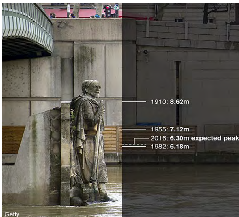
Figure 5 — The statue of the Zouave on the Alma Bridge, Paris, as a flood gauge (Travel France)
