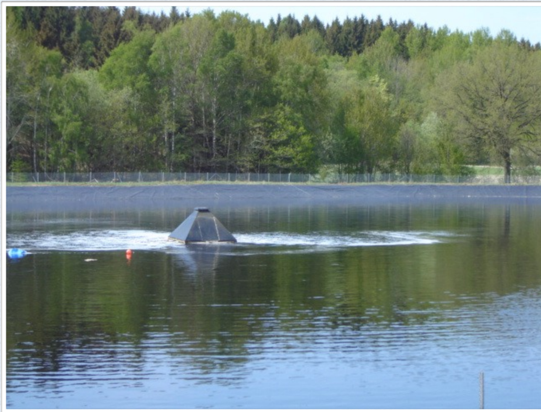
50m 3 /h aerator with a 4 kWh pump from ITT. The pond is 50,000m 3 .
