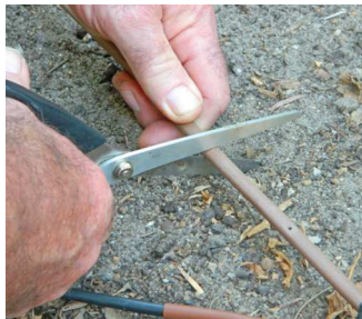
Cut the drip line so that you can connect the Tee
