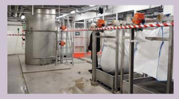
The **Struvia**<sup>™</sup> process is the combination of a crystallization reactor and lamella separator with Veolia's patented Turbomix<sup>™</sup> system, ensuring separation of produced struvite and treated effluent.
