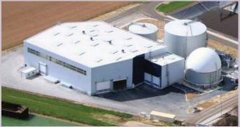
**BIOMET™** is an advanced anaerobic co-digestion process for the conversion of high strength and municipal organic waste to bioenergy and biofertilizer.
