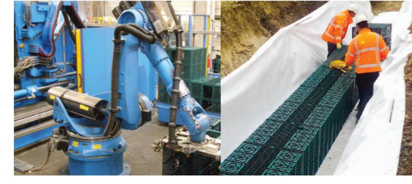
tions of its top quality block at 6.9m below ground level, with over 4m of cover material. And all of that is achieved with a minimum 50-year design life, in accordance with the CIRIA C680 industry standard for structural design of modular geocellular drainage tanks.
