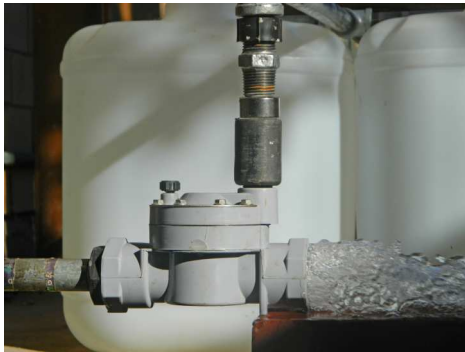
When the magnet is in the low position, the magnet lifts the plunger inside the solenoid and opens the valve
