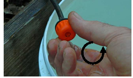
If the volume in the measuring container is more than the dripper control volume, turn the control dripper anticlockwise to increase the flow rate of the control dripper.
