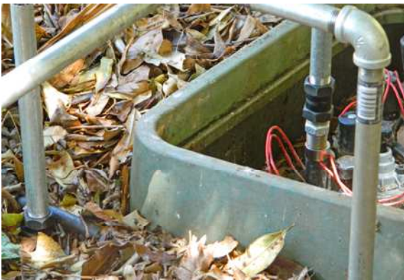
Water slowly evaporates from the evaporator until the weight of the water in the evaporator is light enough for the magnet to fall from the high position to the low position
