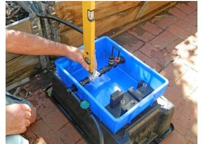
Use a spirit level to ensure that the float shaft is vertical
