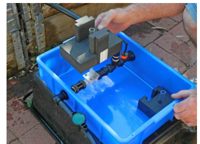
Slide the float over the float shaft
