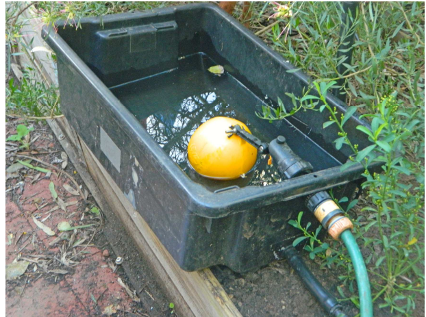
Float valve mounted inside the container
