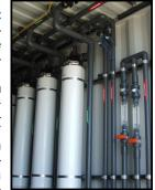
bly strong and chemical resistant. The DLXM membrane modules filter from the outside of the fiber to the inside
