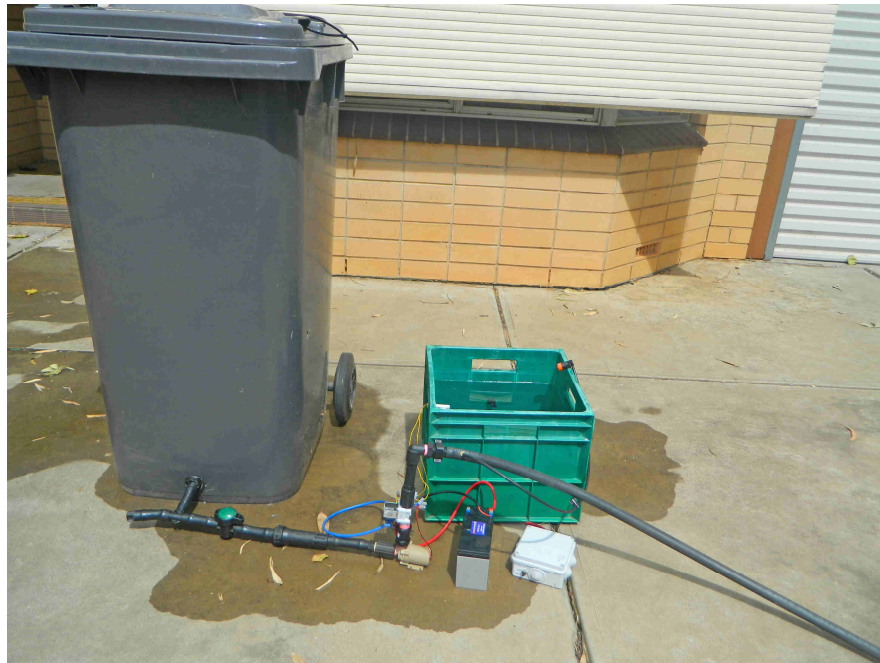
Water in the wheelie bin is used to automatically irrigate all of the garden beds using a Measured Irrigation Controller made from the Kerbside Stormwater Recycling Kit.
