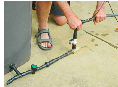
Disconnect the outlet pipe
