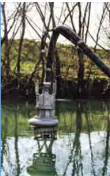
THY85A: canal dredging operation (Italy).
