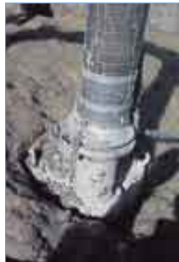
THY24: mud removal from decanting basins (Italy).
