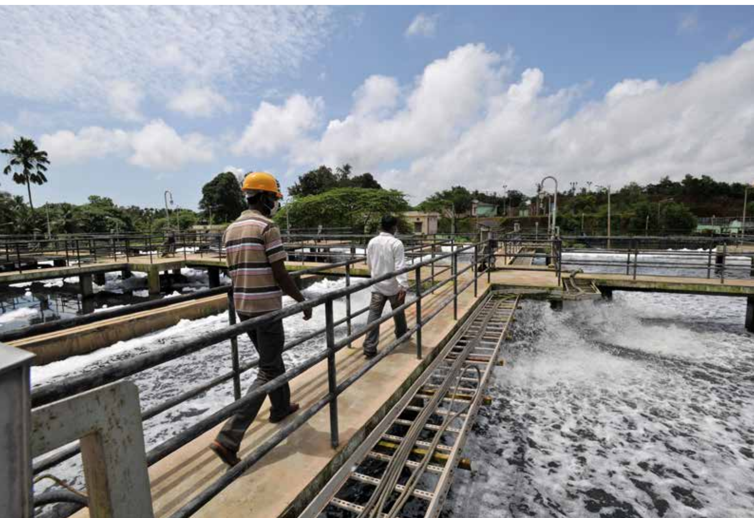
Sewage treatment plant in Kavoor, Mangalore (India) Photo: © Asian Development Bank
