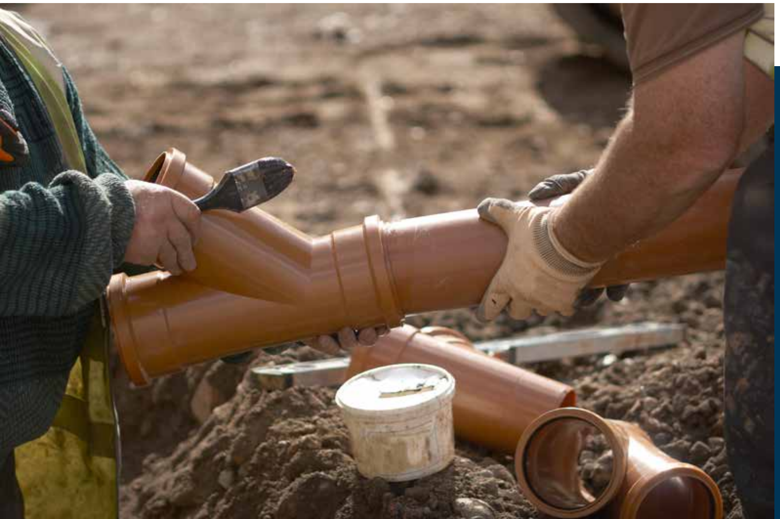
Builder laying sewage pipe on site Photo: © iStock.com/ezza116
