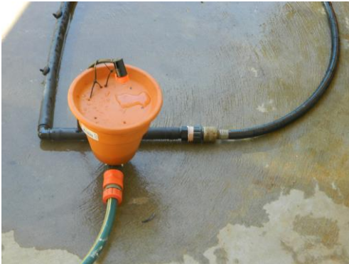
Connect the water supply to the valve inlet and connect the irrigation application to the 19 mm poly pipe
