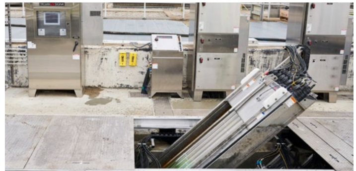
This TrojanUVSigna installation can treat 20 MGD (875 l/s) in only 250 ft 2 (23 m 2 ).
