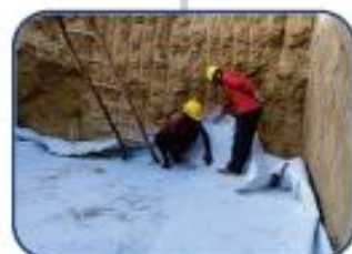
Laying & Cutting of Geotextile
