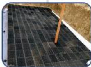
Assembly of Rainmaxx™ Tank
