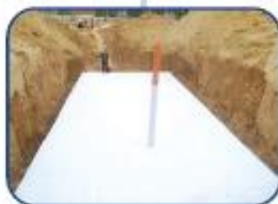
Wrapping of Geotextile
