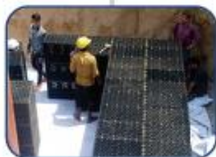
Laying of Rainmaxx™ Modules
