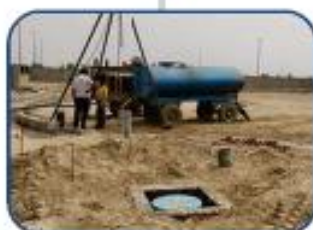
Cleaning of Recharge Well
