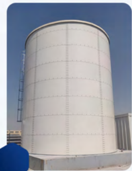
Fusion Bond Epoxy Tanks
