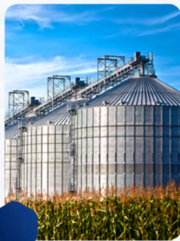
Grain Storage Silos
