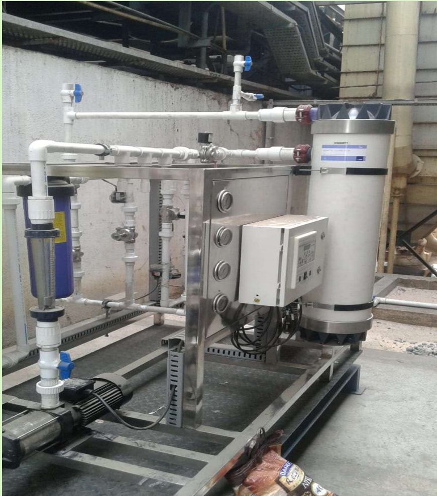
BASF INDIA , TURBHE 1000 LPH ULTRA FILTRATION PLANT
