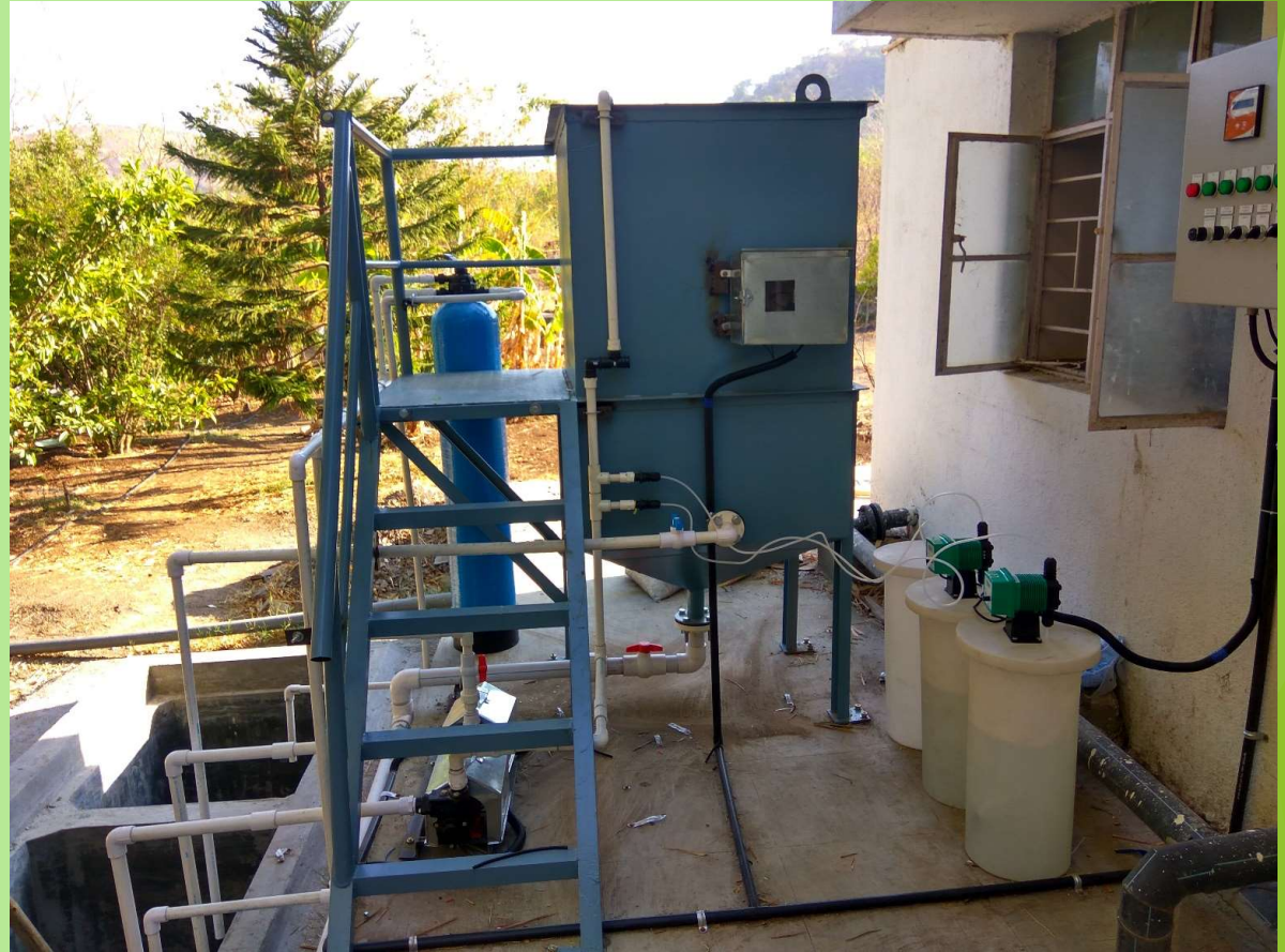
KNOWCHEM LABORATORIES- PUNE 2 KLD ETP
