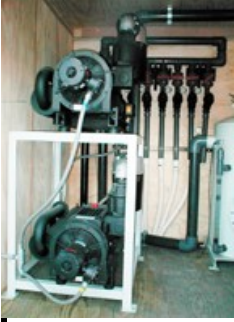
Claw Pumps Two 325 cfm stacked
