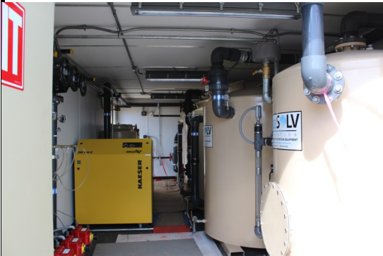
dry running and has extremely low maintenance 200 cfm DPE with a PD Blower
