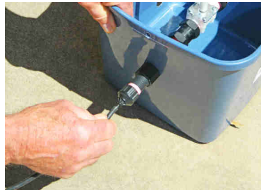
Use a tube to deliver water from the outlet pipe on the bucket to the inlet pipe of the wicking bed
