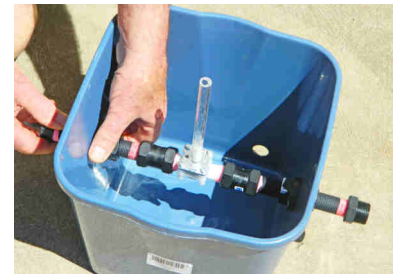
Tighten the internal back nuts against the external round plastic nuts
