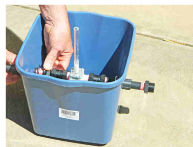
Insert the outlet pipe through the other hole and reattach the washer and the back nut
