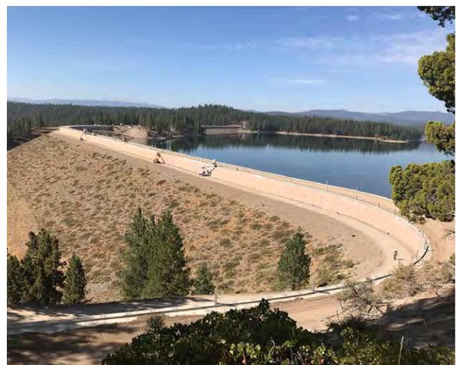
Downstream face of Stampede Dam, California, showing the 11.5-foot-high crest raise (Reclamation).
