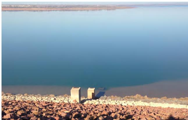
Foss Reservoir in Oklahoma taken in March 2015, at the end of the recent drought. Picture shows three intakes, two of which are dry. The top of the third intake can just be seen through about six inches of water, signaling a potential need to take emergency action to access the lowest pools of the reservoir.
