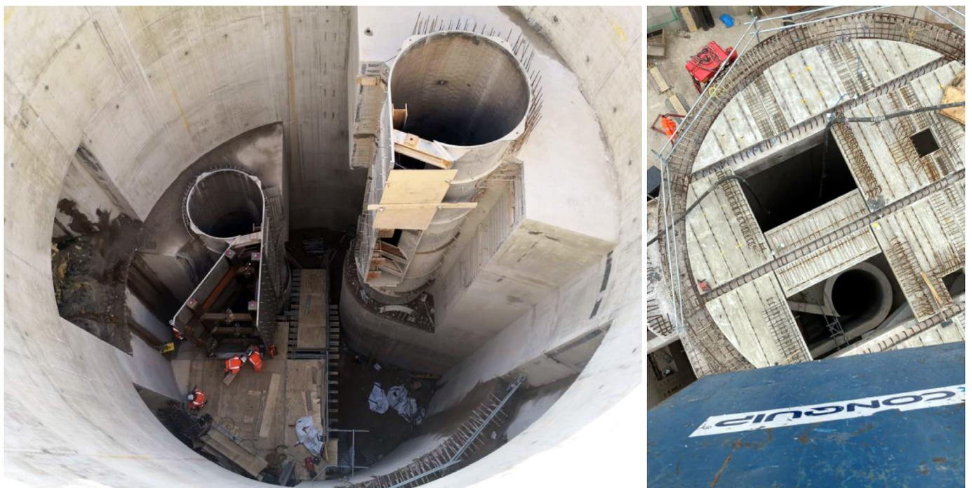
Figure 3 | Examples of steel lining of TTT tangential vortex intake during construction (left) and tangential intake with concrete encasement prior to installation of shaft covers (right).
