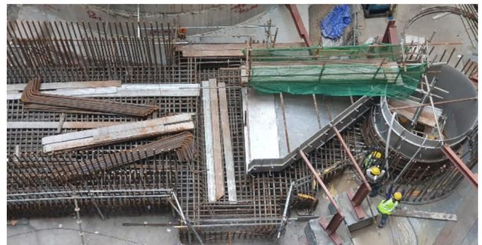
Figure 2 | Vortex generator and drop structure under construction.
