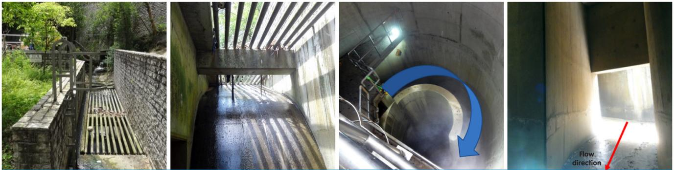
Figure 6 | Example of compact tangential vortex intake in HKWDT system.
