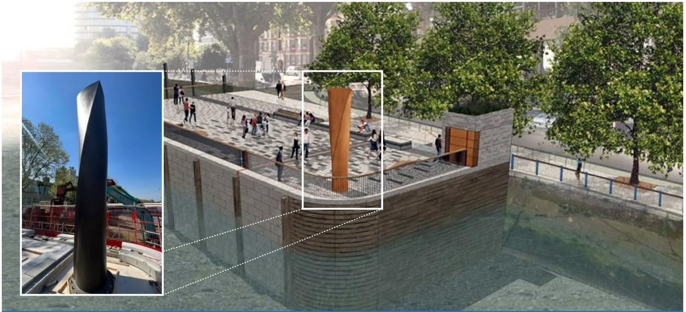
**Figure 7** | SDG15 – Enhancing life on land. New river-shore developments have provided a unique opportunity to provide seven new landscaped areas above the drop structures developed in the Thames Tideway Project, including an artistic drop structure ventilation column resembling the top surface of the vortex flow passing down the drop structure below the area. (Courtesy of Thames Tideway).
