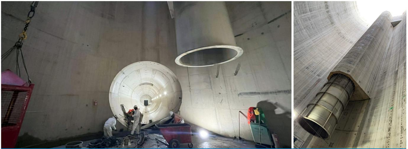
**Figure 4** | Examples of TTT drop shafts during construction with base of vortex drop tube and horizontal deaeration tunnel visible (Left) and full height of a finished vortex drop (right).
