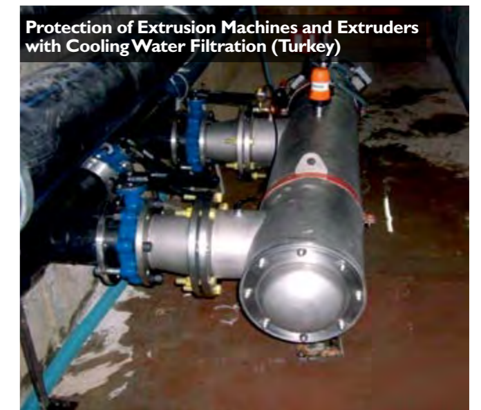
Plastic Industry, Cooling Water Filtration for Extrusion & Extruder (Turkey)
