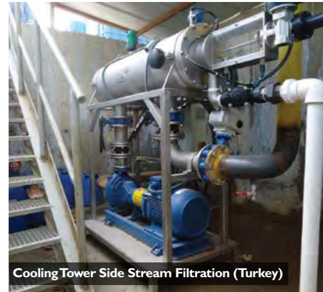
Steel Industry, Cooling Tower Filtration (Turkey)
