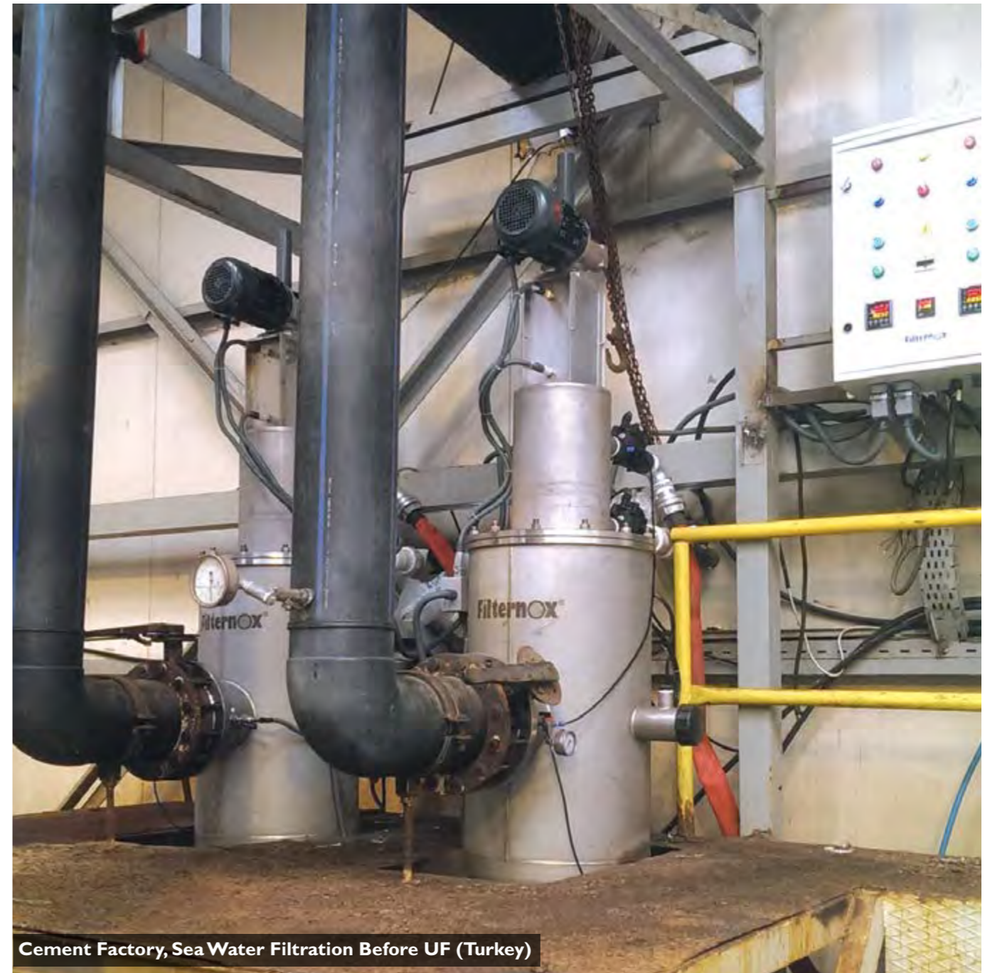
Two Stage Filtration of Sea Water Before Heat Exchangers (Turkey)
