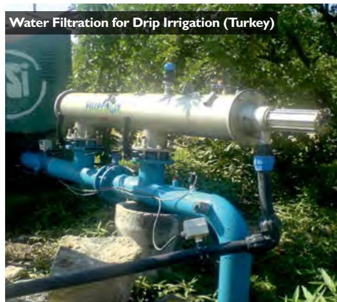
Water Filtration for Drip Irrigation (Turkey)
