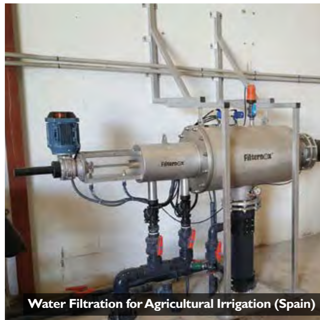
Water Filtration for Agricultural Irrigation (Spain)
