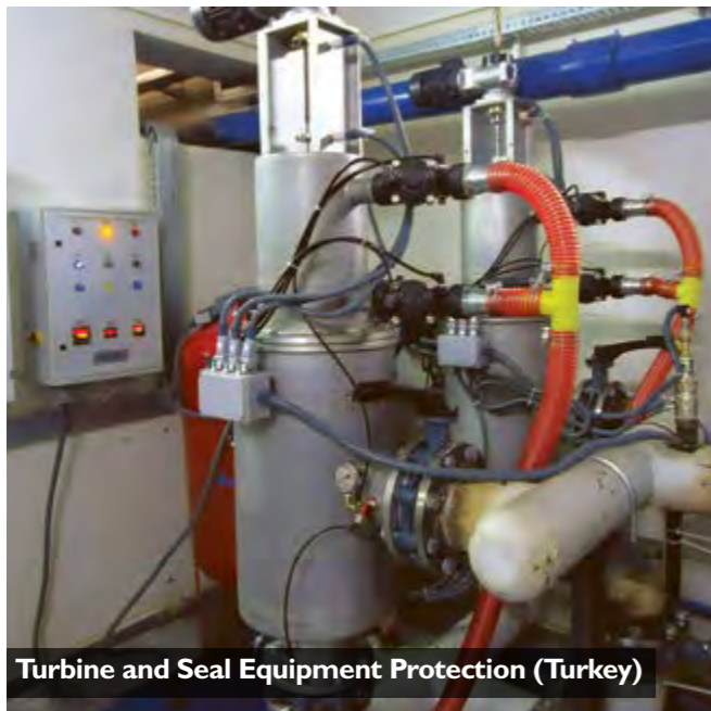
Power Generation Plant, River Water Filtration (Turkey)
