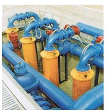
VERTICALLY-MOUNTED SUBMERSIBLE PUMPS installed inside metal barrels eliminate the need for mid-level storage tank.
