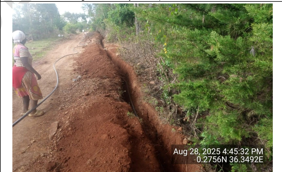
4. Pipe trenching, pipe layong and backfilling
