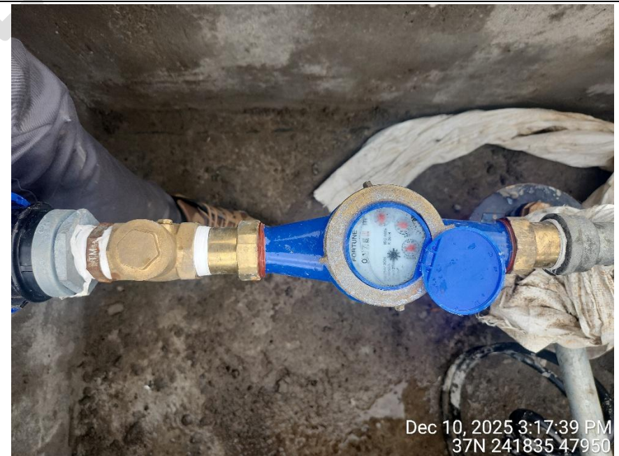
12. BH chamber and meter installation
