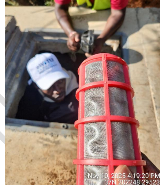
10. Chamber outlet Y-Strainer
