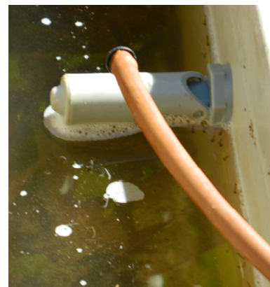
Horizontal float switch mounted on the side of the evaporator.
