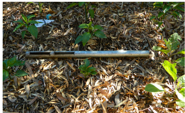
An angle grinder is used to make some slots in a length of steel pipe
