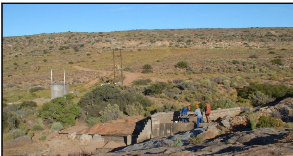
Figure 36 - Sand filter with injection and abstraction borehole (pump house) in the background (Murray, 2008).
