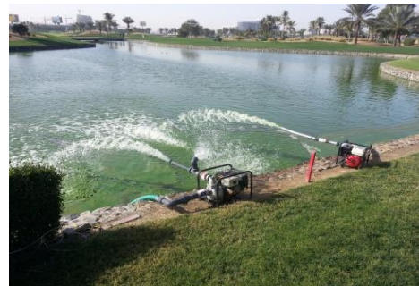
Embankment Magnetised circulation pumps
