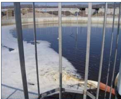
Before: (using a traditional venture aerator)
