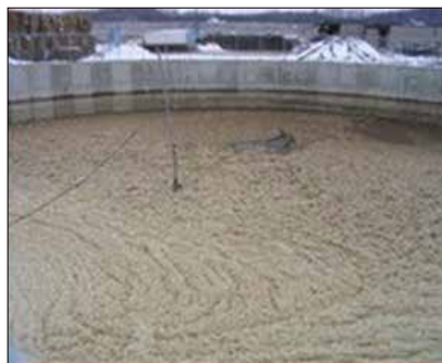
After: (using SAR Aerator after 30 days of operation)
