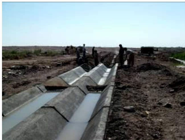
Photos showing different stages of construction of the new canals for conveyance of the Eisavieh and Najmieh Qanats water. Top: preparation of the foundation, Middle: cutting out the x-section, Bottom: lining in progress.
