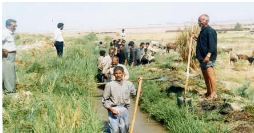
Members of Water Users Group of the twin qanats of Eisavieh and Najmieh during cleaning operations of the conveyance canal (May 2004). Concrete lining of this channel was included in the UNDP project. All members of the WUG requested that an independent canal be built for each qanat (unlike the original situation where one canal conveyed water of both qanats).
