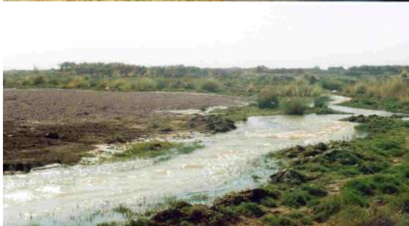
The twin qanats of Eisavieh and Najmieh and the conveyance canal downstream from their mouth. Lots of water was lost along the 4-km course of the channel due to seepage into the ground.
