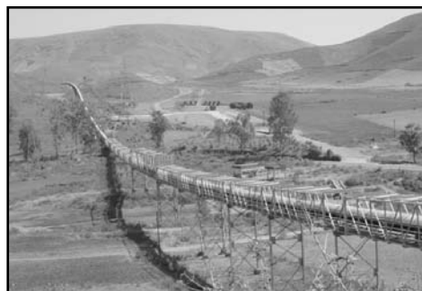
NALCO mine to refinery conveyor belt, Damanjodi.
