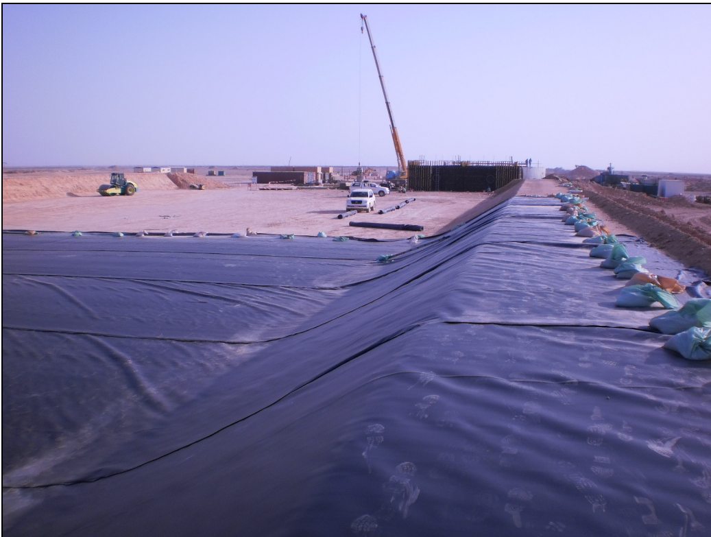
Installation of a HDPE liner
