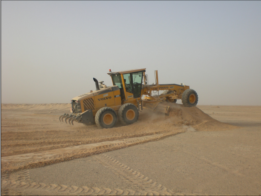
Start of the levelling works on site
