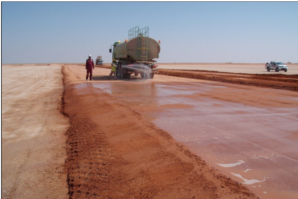
Installation of a mineral sealing layer
